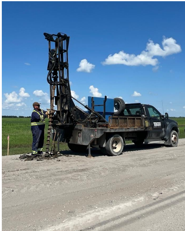
Figure 2941. Drill rig at Winkler Site
