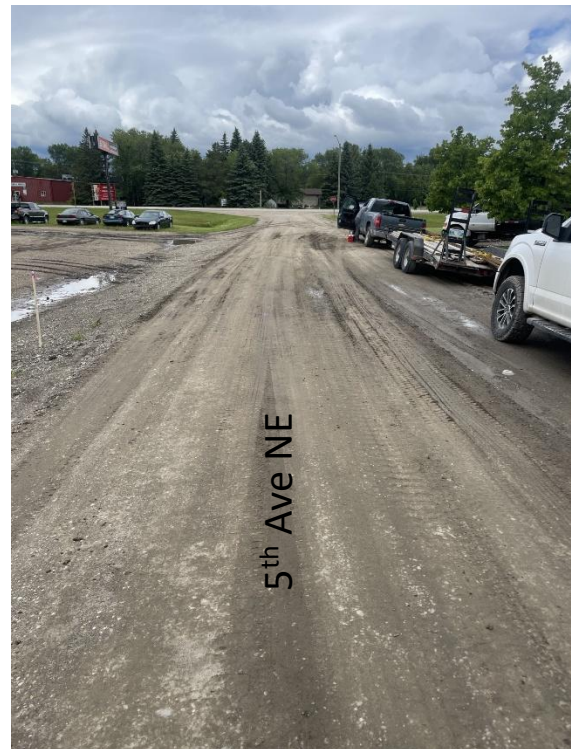
Figure 257. Rutting in problem area, view W
