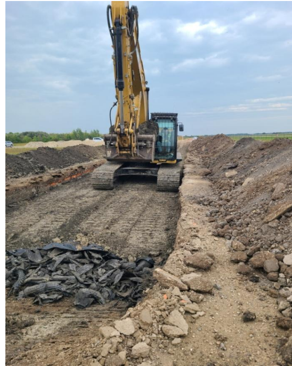
Figure 2381. Placing first lift of soil cover over TDA (photo courtesy of P. Schroedter)
