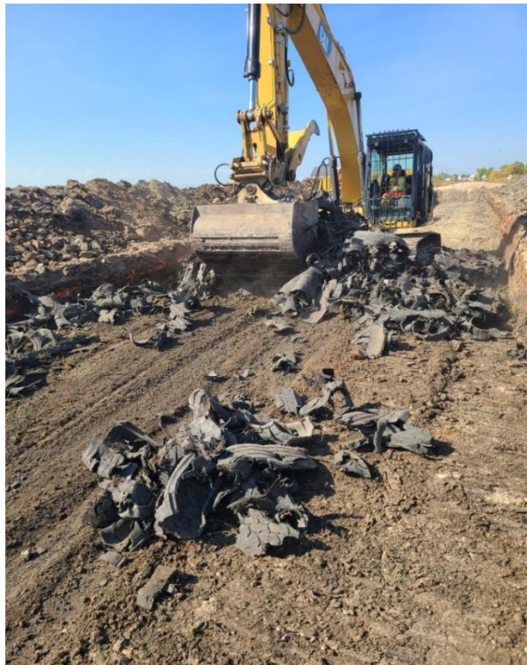
Figure 2221. Placing first lift of TDA in cut (photo courtesy of P. Schroedter)
